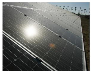
**Glint:** Also known as specular reflection, the direct reflection of the sun on the surface of the solar module can produce glint. This is the primary source of concern regarding visual distraction, and SunEdison modules with ARC glass are no more reflective than water and half as reflective as car windshields.
