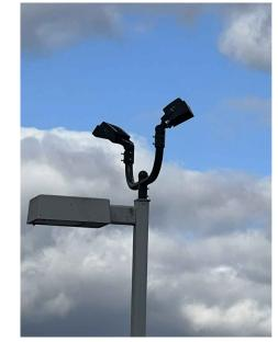
CUSTOM SHIELDS SHOWN **INSTALLED ON 75 LED SERIES** FLOOD LIGHTS (FLD)
