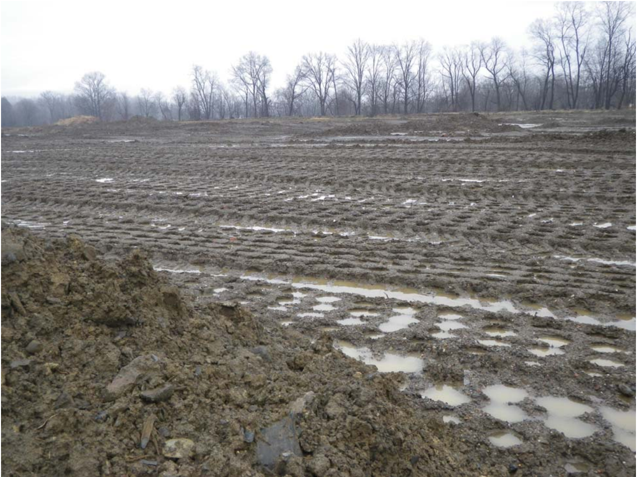
The south-central area of the site where fill material has been placed, spread and compacted using a Sheepsfoot roller.
